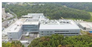
Completed construction of the new Sanda Factory (2020)
