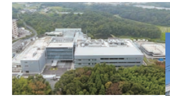
Construction of the new Sanda Factory (2020)
