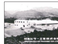
Construction of the Sanda Factory in Sanda, Hyogo, Japan (1967)
