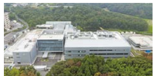
Completed construction of the new Sanda Factory (2020)
