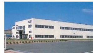
Completed construction of the Fukuchiyama Factory (currently Fukuchiyama Factory No. 1) in Fukuchiyama, Kyoto Prefecture, Japan (1989)
