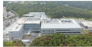
Completed construction of the new Sanda Factory (2020)
