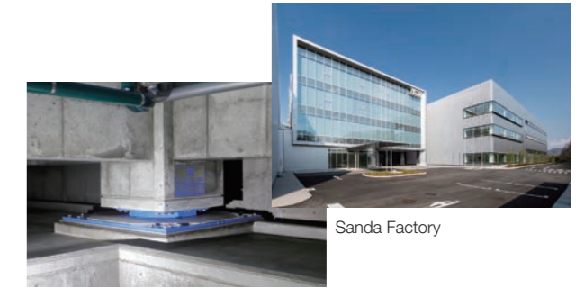
Seismic isolator / Slide bearing
