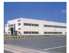
Construction of the Fukuchiyama Factory (currently Fukuchiyama Office) in Fukuchiyama, Kyoto Prefecture, Japan (1989)
