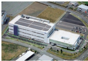
Construction of the Kyushu Factory in Koshi, Kumamoto Prefecture, Japan (2004)
