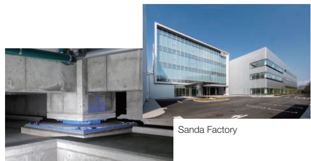
Seismic isolator / Slide bearing
