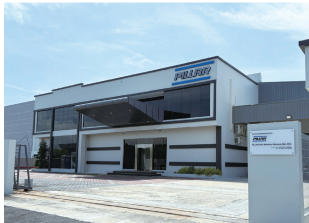
PILLAR Seal Solutions Malaysia Sdn. Bhd
