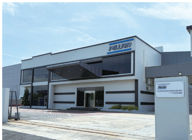
PILLAR Seal Solutions Malaysia Sdn. Bhd
