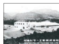
Completed construction of the Sanda Factory in Sanda, Hyogo, Japan (1967)
