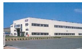
Completed construction of the Fukuchiyama Factory (currently Fukuchiyama Factory No. 1) in Fukuchiyama, Kyoto Prefecture, Japan (1989)
