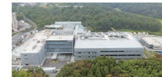
Completed construction of the new Sanda Factory (2020)
