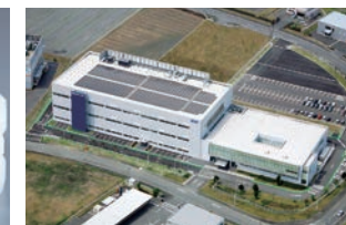
Completed construction of the Kyushu Factory in Koshi, Kumamoto Prefecture, Japan (2004)
