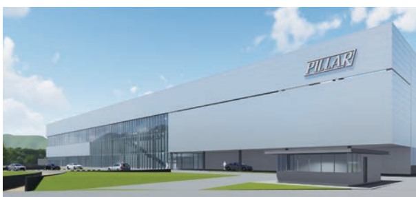
Illustration of completed Fukuchiyama Second Factory
