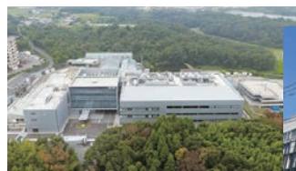
Construction of the new Sanda Factory (2020)
