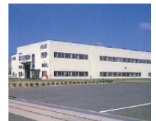
Construction of the Fukuchiyama Factory (currently Fukuchiyama Office) in Fukuchiyama, Kyoto Prefecture, Japan (1989)
