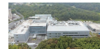
Completed construction of the new Sanda Factory (2020)
